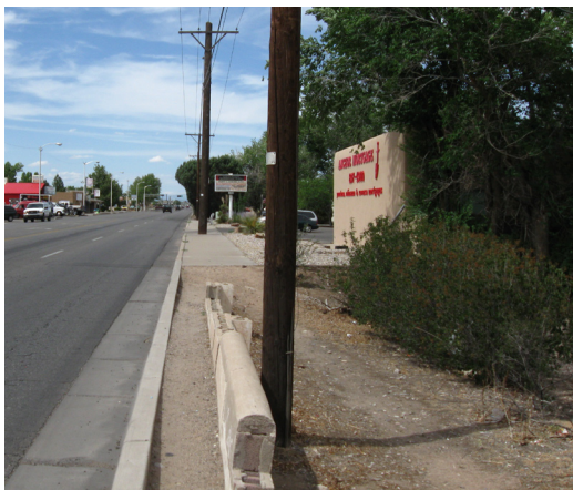
FIGURE 6-6 UNPAVED AND OBSTRUCTED SIDEWALK
